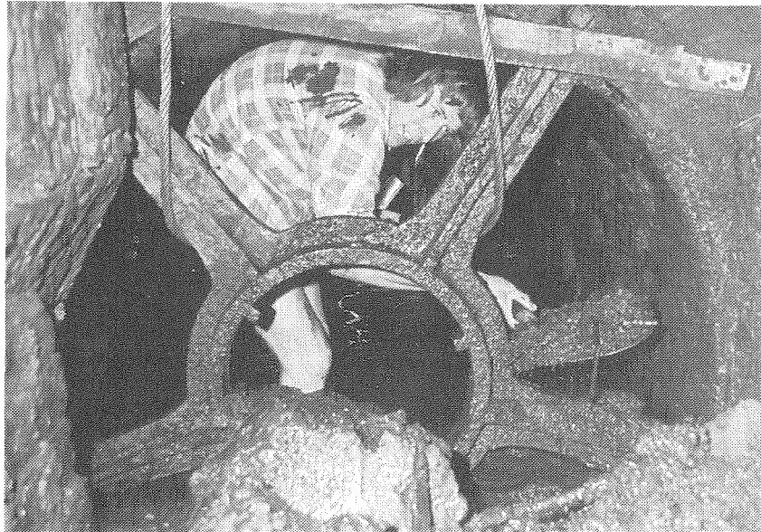
Fig. 4: John Bignell shovelling mud from inside the waterwheel in 1975. Prior to reconstruction, the wheel had become buried in silt and was covered by water. Photograph by Peter Bignell.
