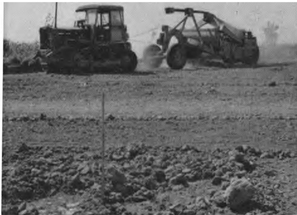
Ground preparation with a scraper and a terracer . (terracer).
